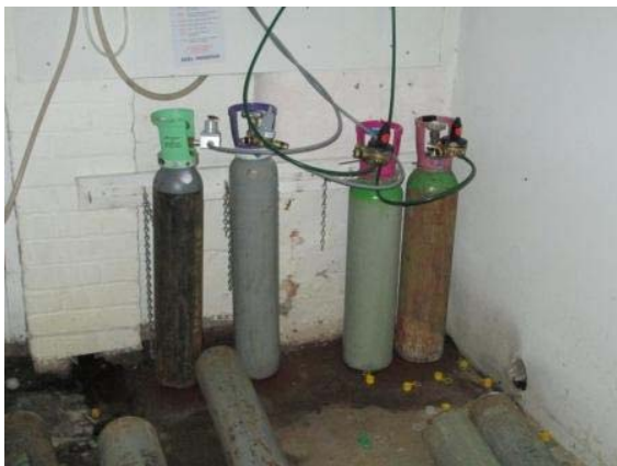
Unchained gas cylinders and an accumulation of rubbish behind the bar
