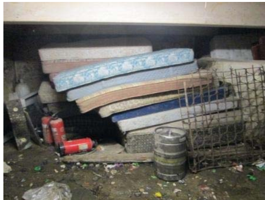
The cellar cooler in a poor state of cleanliness and combustible materials in the cellar
