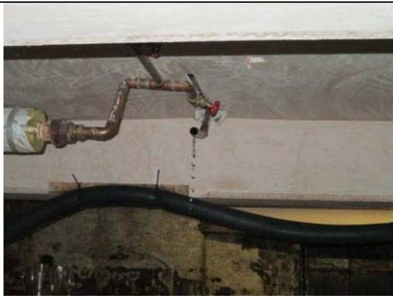
The cellar cooler still in a poor state of cleanliness and leaking water pipe pouring with water resulting in the flooded cellar
