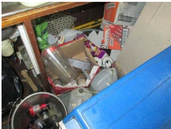
Unchained gas cylinders and an accumulation of rubbish behind the bar
