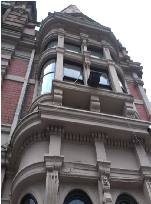
8) Electrical connections to outside lighting that require further investigation.
