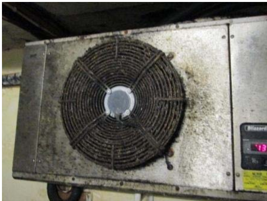
The cellar cooler in a poor state of cleanliness and combustible materials in the cellar
