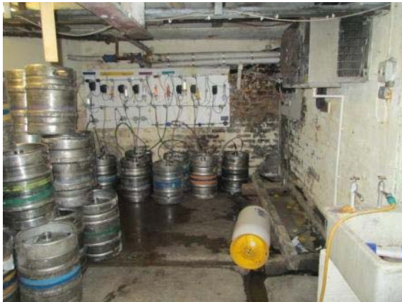
The cellar cooler still in a poor state of cleanliness and leaking water pipe pouring with water resulting in the flooded cellar
