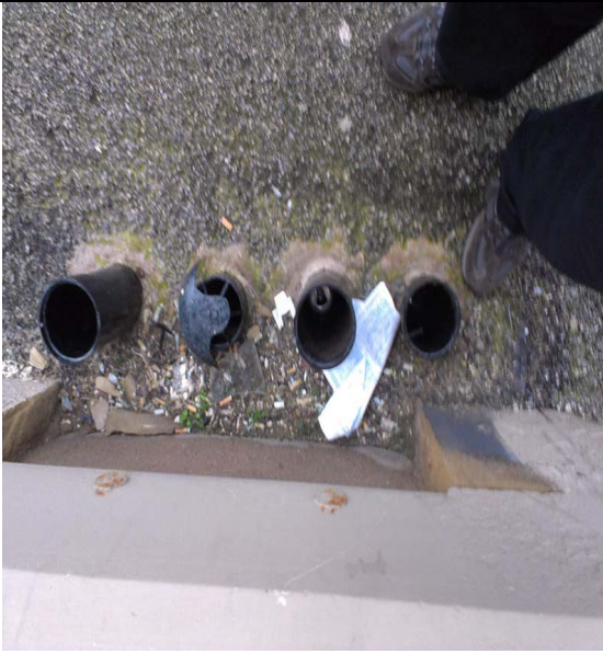
7) Incoming air and flue arrangements that are damaged blocked by cans and debris
