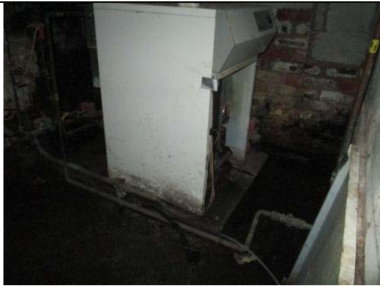
Leaking pipe has flooded the cellar and gas boiler with cover missing
