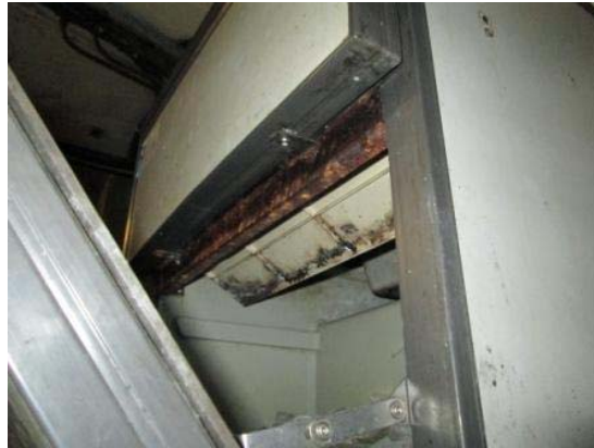
Photographs of the ice machine in poor state of cleanliness and corroded internally
