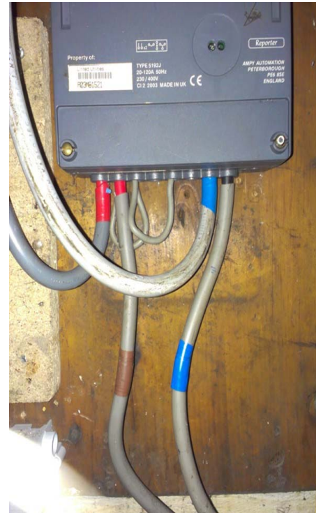
4) Untidy and cluttered cellar area and left the electric meter with seals missing.
