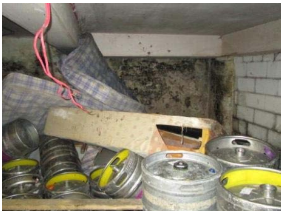
Loose wires to the fire alarm above combustible materials and a leaking water pipe
