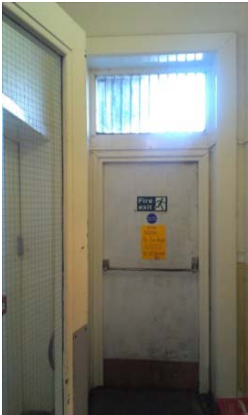
The fire door marked up as a fire escape then the accumulation of rubbish blocking the egress route
