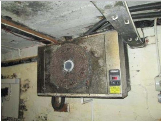
The cellar cooler still in a poor state of cleanliness and leaking water pipe pouring with water resulting in the flooded cellar
