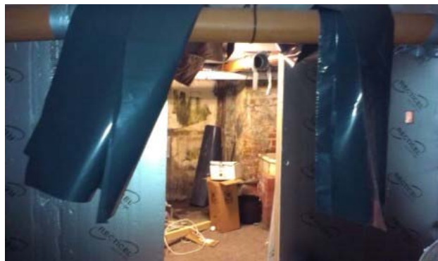
The remnants of drug cultivation equipment is still evident in the cellar, the photographs showing the wall insulation and ducting still present along with the dangerous electrics.
