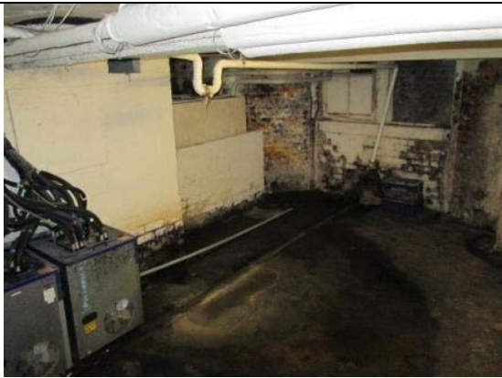
Leaking pipe has flooded the cellar and gas boiler with cover missing
