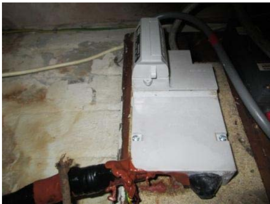
Electricity meter has missing security seals indicating possible evidence of meter tampering
