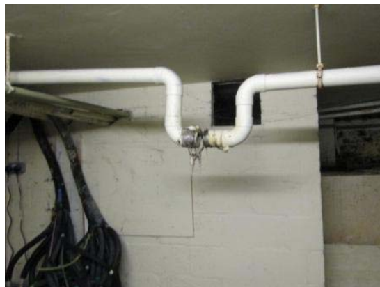
Loose wires to the fire alarm above combustible materials and a leaking water pipe
