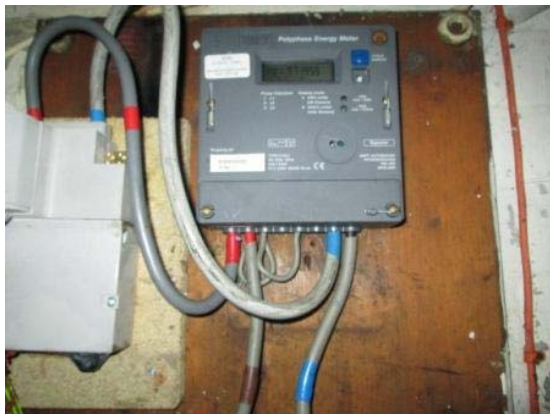
Electricity meter has missing security seals indicating possible evidence of meter tampering
