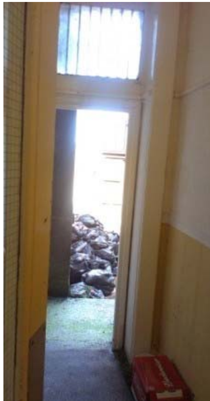
The fire door marked up as a fire escape then the accumulation of rubbish blocking the egress route
